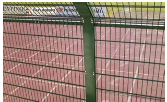
Omega post 120x60x30x3 mm section
